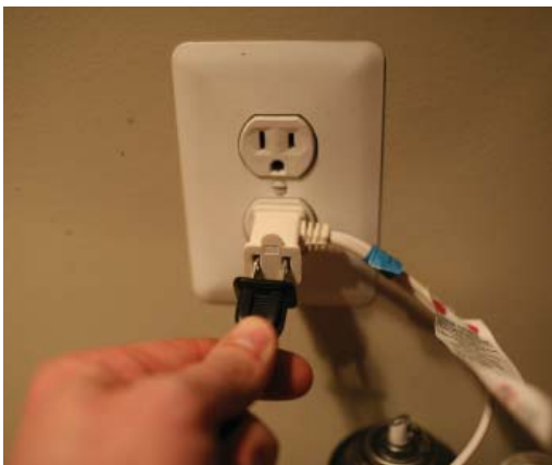
Insert plug into the on/off switch extension cord (provided), that is in turn, plugged into a 120vac outlet (Figure 2)
